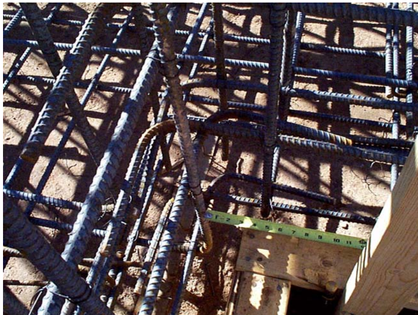
Figure 1. Flexural and tension steel reinforcement at a wall-to-wall corner.
